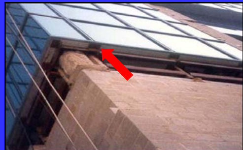
TYPE I DESIGN--CURTAIN WALL (ALSO CALLED SAFING GAP)
