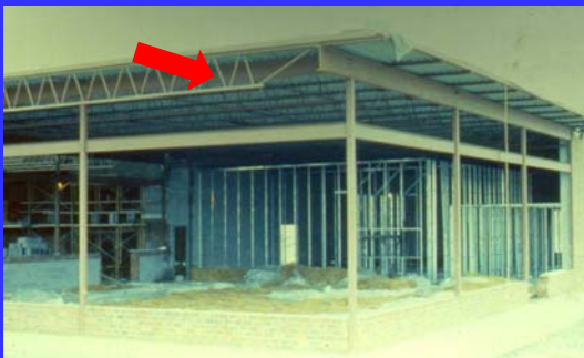
TYPE II DESIGN--UNPROTECTED STEEL FRAME WITH TRUSS
