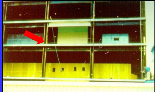
TYPE II DESIGN--STEEL WITH COLUMNS FOR SUPPORT
