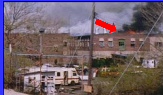
TYPE III DESIGN--ROOF COVERING ADDS TO FUEL LOAD
