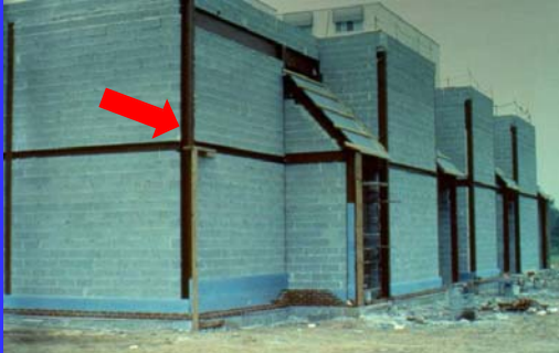
TYPE II DESIGN--CINDER BLOCK WITH METAL FRAME SUPPORT
