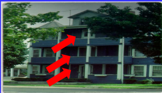
TYPE V DESIGN--BALLOON FRAME (cont'd)
