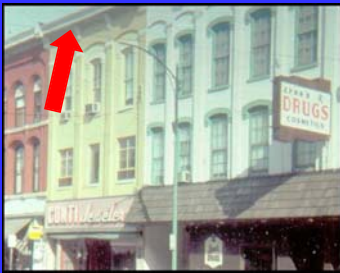
TYPE III DESIGN--WOODEN CORNICE
