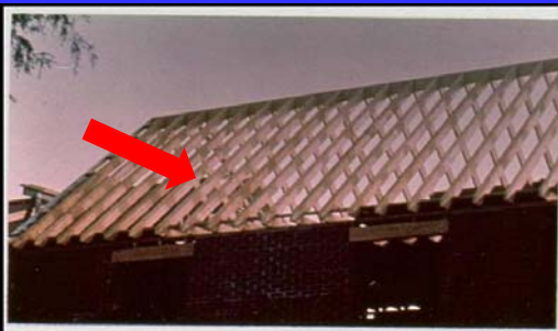
TYPE III DESIGN--RIDGE POLE SUPPORTS MAIN ROOF
