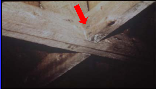
TYPE III DESIGN--TOE-NAILED JOINTS
