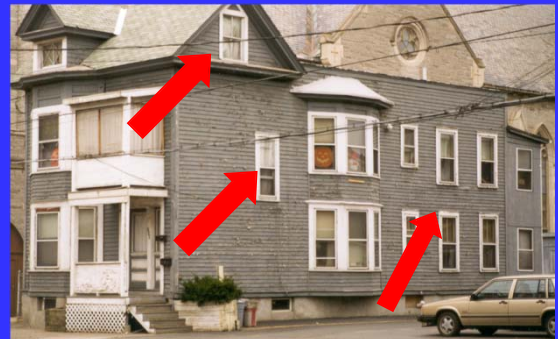
TYPE V DESIGN--BALLOON FRAME
