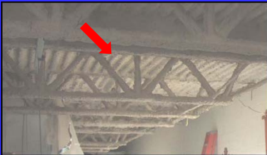
TYPE I DESIGN--SPRAY ON FIRE PROTECTION--STEEL TRUSS
