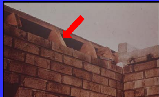
TYPE III DESIGN--FIRE CUT
