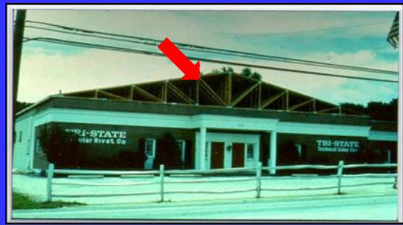
TYPE III DESIGN--TRUSS ROOF SUPPORTS
