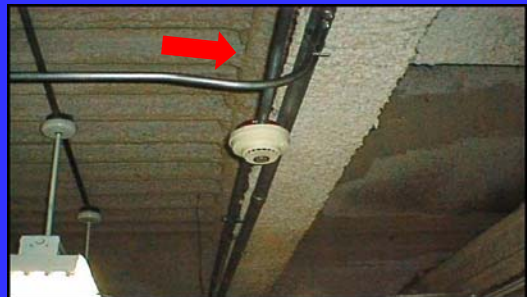
TYPE I DESIGN--SPRAY ON FIRE PROTECTION--STEEL JOIST AND CEILING
